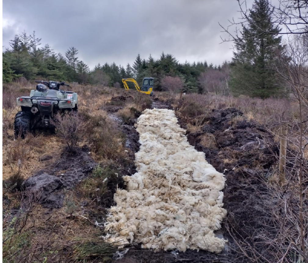
A popular coastal path at Kilmarie on Skye, provided an ideal opportunity to try a sustainable path repair technique that used locally-sourced wool
