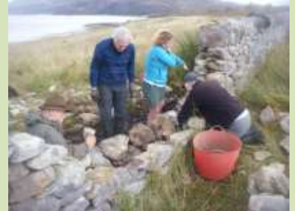
Drystone dyking on Isle Martin
