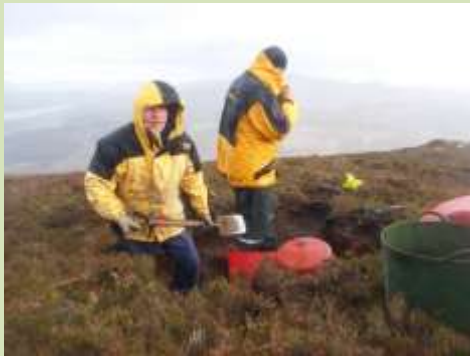
Digging a borrow pit on East Schiehallion
