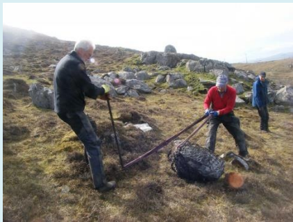
Path work on Huishinis to Cravadale path
