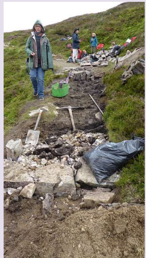
Rebuilding the path on East Schiehallion
