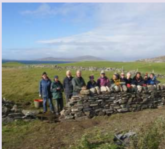
Proud volunteers behind a dyke they are building on West Harris
